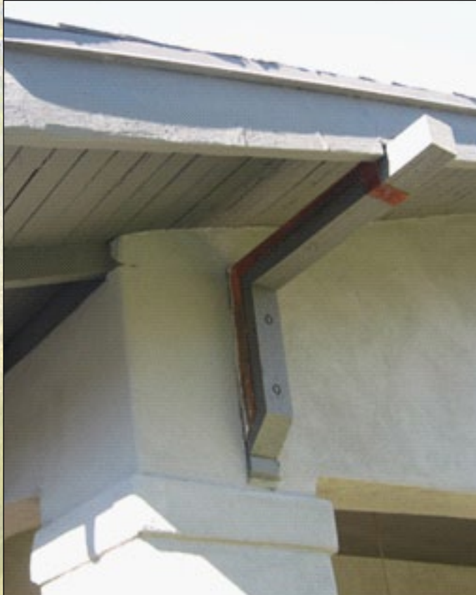
Overhang Bracket: Pressure-treated Wood and Steel
